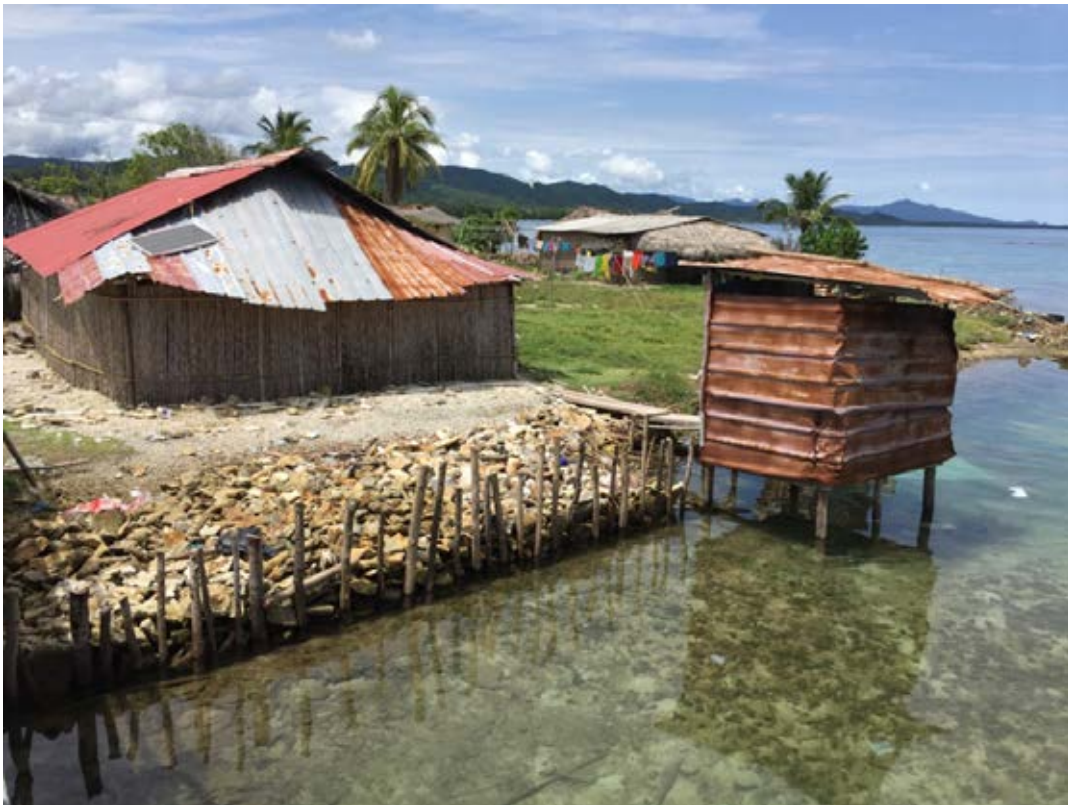
Landfilling in Niadub (Isla Diablo). This is the typical way landfilling is done in Gunayala to expand the area of the islands. The structure on the right is the typical latrine used on Gunayala's islands. Photo by Carlos Arenas.
