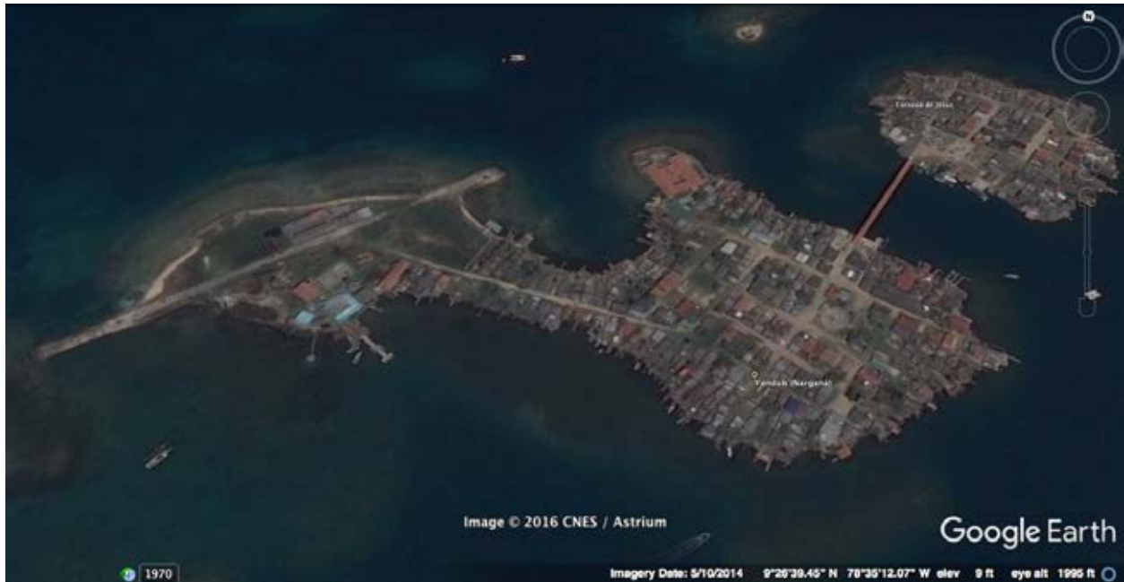
Google Earth's image of Yandub (Narganá) and Corazón de Jesús, and the bridge that connects the two islands.
